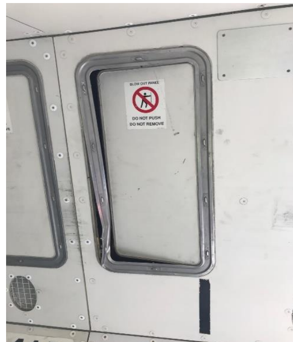
Blow-out panel frame distorted
