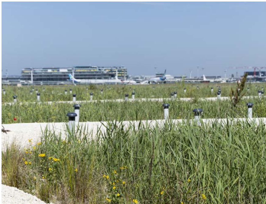
Filtering marshes for winterizing products (glycol), Stormwater treatment system (STP) at Orly. © Zoo studio/ADP
