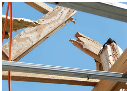
Figure 2 : Section insuffisante
